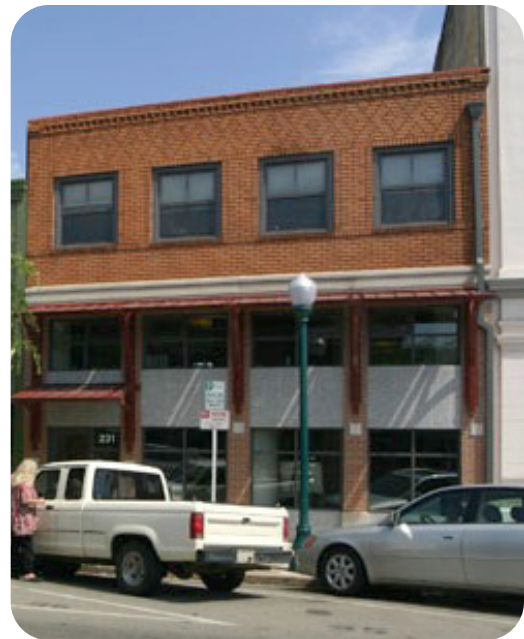
Land Architecture Building on Vernon Street after renovation
